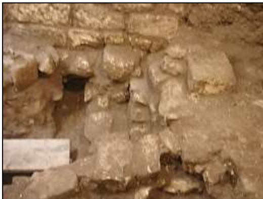
Figure.8:(a) An image showing foundation construction with rubble stone, Ahmed Katkhuda EL-Razaz, (ARCE conservation project. Historical Cairo.
